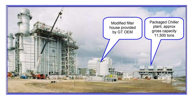
This figure shows a S207FA in Texas, USA, with a nominal power rating of 633 MW. This plant was originally designed for both chilling and high rates of supplemental firing. In summer operations, the chiller capacity is dispatched before the firing capacity, which is held in reserve for the hottest days only when economic dispatch is made possible. Two TAS "F-50" chiller systems are shown on the right side of the picture. Combined net coil demand is approximately 10,500 tons (refrigeration).
