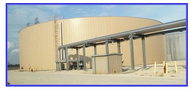
Pictured below is a 6+ million gallon tank installed in 1999 for a partial storage design involving 3 W501D5s GTs.
